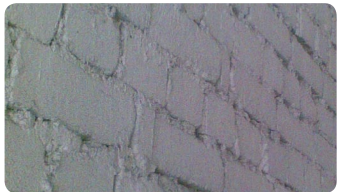
Fig. 2 Dust is captured in open grouting.
